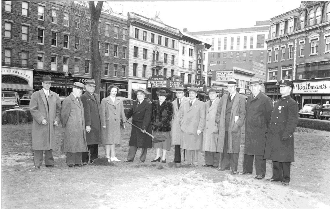
Advocate—Seaf Construction of the Stamford Service Roll started this morning with Department of Service workmen, under the supervision of Councilman Ralph Rich, member of the Service Roll Committee, making the required excavation. A concrete foundation will be constructed. The work of preparing the slats which will bear the names of Stamford men and women in service is also being pushed as is the millwork for the monument at Stamford Trade School under the direction of Frank Laney. The committee on names, Col. James Wild, Kingsley Gillespie and Samuel Morrell, is seeking the names of all Stamford people in service at any time during the current conflict. Present in Central Park yesterday as ground was broken for the Service Roll were: Left to right—Dr. Charles E. Frange, Deputy Commissioner of Finance Frank C. Langley, Commissioner of Finance Frank T. Slavin, Mrs. Bindley Gillespie, Mayor Charles E. Moore, shown wielding the spade; Mrs. David Waterbury, sr., Corporation Counsel Charles N. Wexler, Kingsley Gillespie, City Engineer Leon C. Tuttle, Lieut. Col. James H. Wild and Patrolman Asa W. Scanlon, veteran of the World War I.
